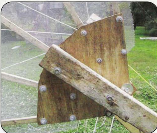
Photo B. The struts are attached to a square plywood center with two bolts.
